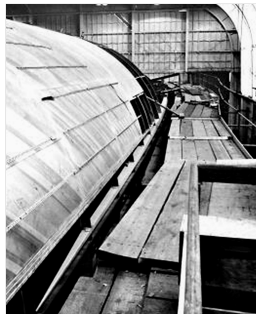
Top to Bottom: Hughes Aircraft workers assembling one of the H-4’s eight engine nacelles from Wisconsin plywood. Much of the wood was held in place with temporary nails or rivets while the glue set. Hughes workers used more than eight tons of nails building the H-4.
